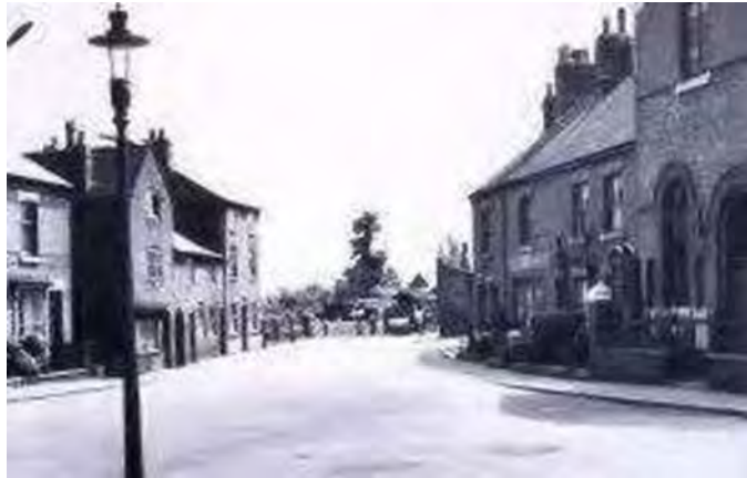
Figure 12: Old view along Church Street
